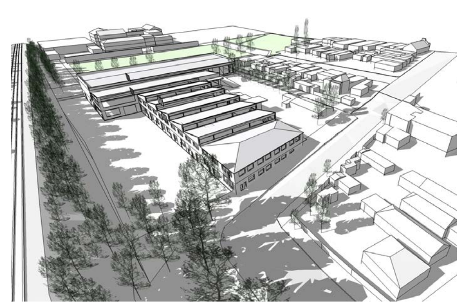
Existing situation - 22 MARCH - 3 pm
